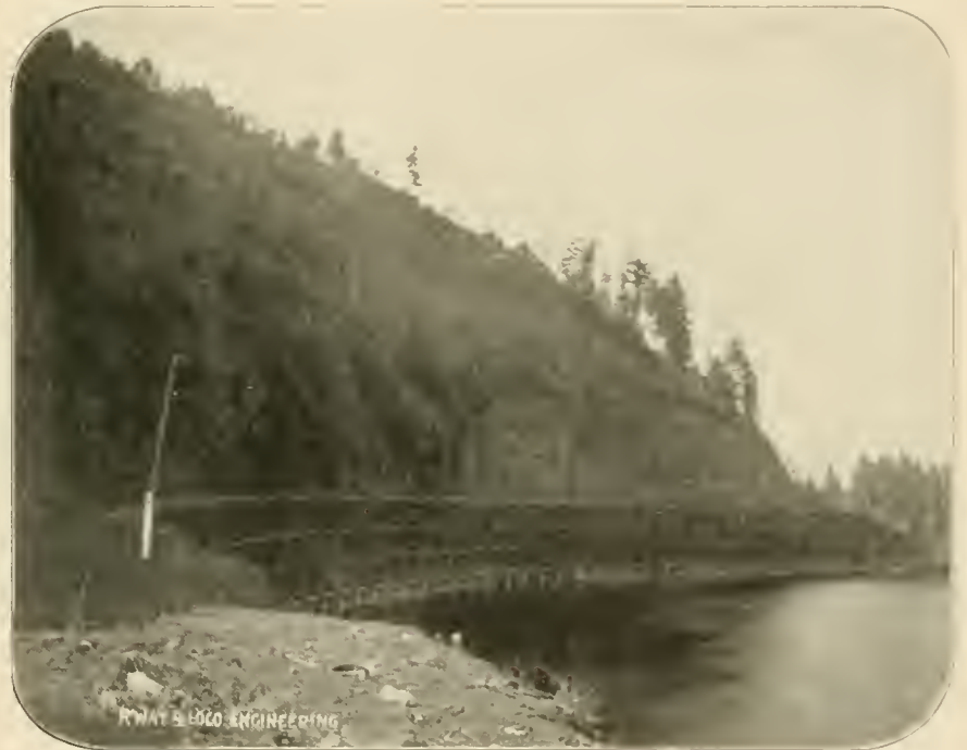
ELK ROCK TRESTLE, NEAR PORTLAND, ORE.
